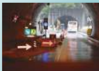
Service and utility tunnels, construction sites
